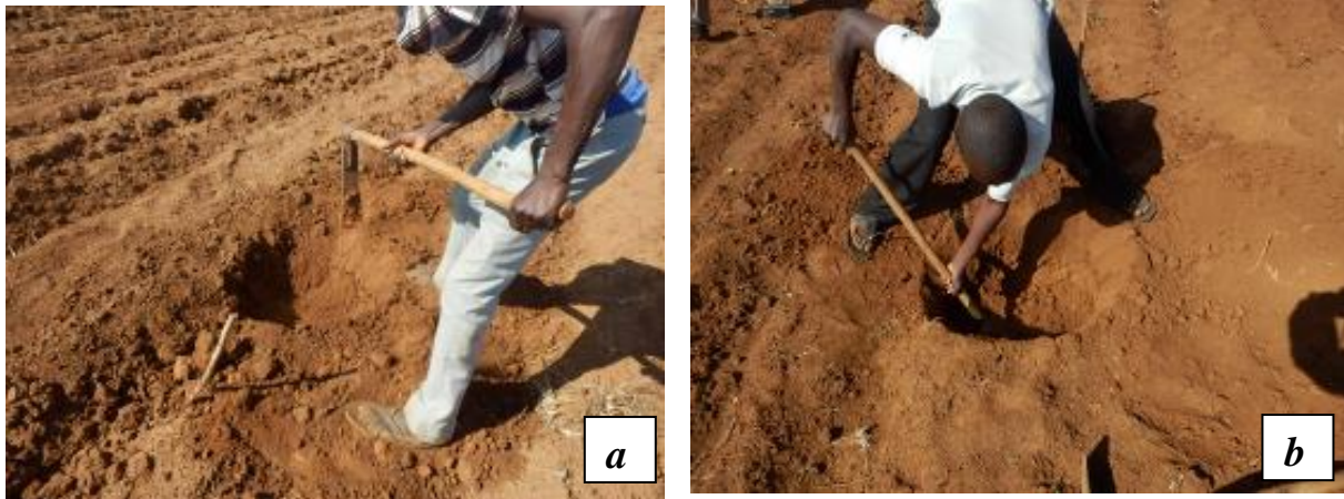
Plate 19: The pitting process: (a) Digging up the pit and (b) refilling the pit
